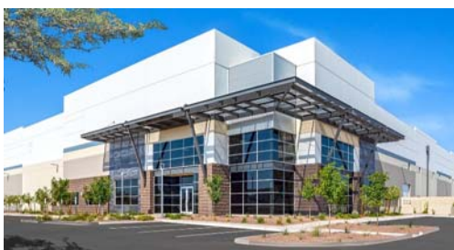
First Park PV303 Building B | Goodyear, AZ
