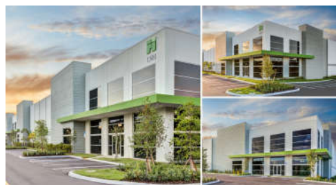
First Cypress Creek Commerce Center | Fort Lauderdale, FL
