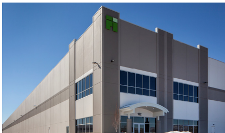
First Logistics Center @ I-78/81 – Building B
