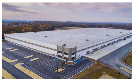
First Logistics Center @ I-78/81 – Building A
