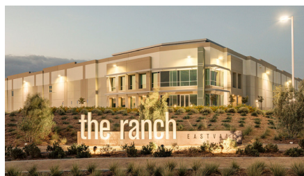
The Ranch by First Industrial – Building 5
