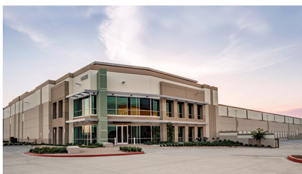
The Ranch by First Industrial – Building 3
