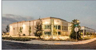
The Ranch by First Industrial – Building I 49,571 SF
