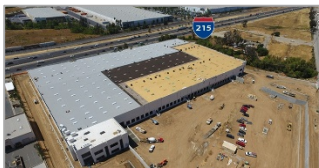
First Sycamore 215 Logistics Center 242,580 SF
