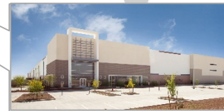
First Park @ PV 303 618,350 SF
