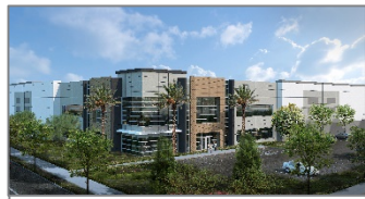
First Perry Logistics Center 239,950 SF Estimated Completion: 4Q19
