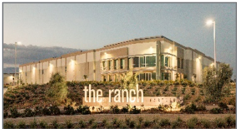
The Ranch by First Industrial - Building V 220,707 SF
