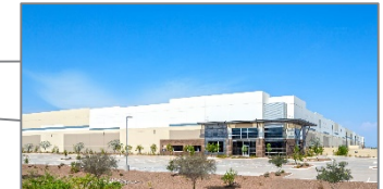
First Park @ PV 303 - Building B 643,798 SF
