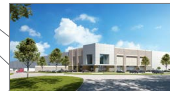
First Mountain Creek - BTS 863,328 SF Estimated Completion: 4Q19
