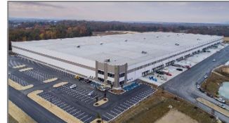
First Logistics Center @ I-78/81 - Bldg A 738,720 SF
