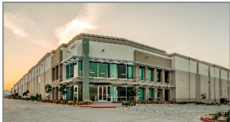
The Ranch by First Industrial - Building II 155,742 SF
