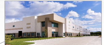
First Park 94 - Building II 602,348 SF
