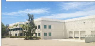
1445 Engineer St 99,307 SF
