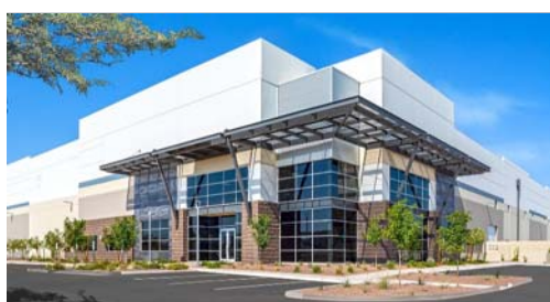
First Park PV303 Building B | Goodyear, AZ
