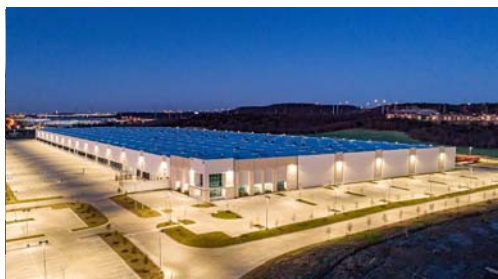
Mountain Creek Distribution Center | Dallas, TX
