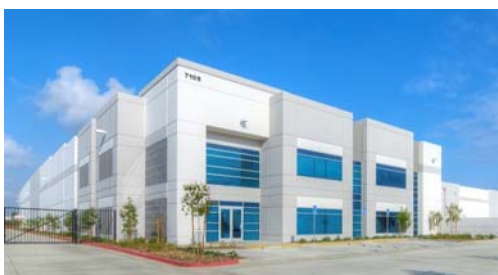
First Sycamore 215 Logistics Center | Riverside, CA
