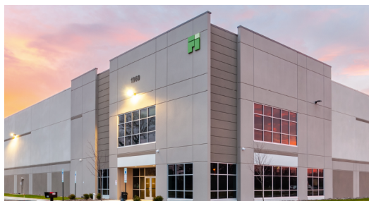
First Lehigh Logistics Center Allentown, PA
