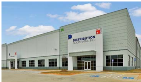
First Park McDonough-BTS | McDonough, GA
