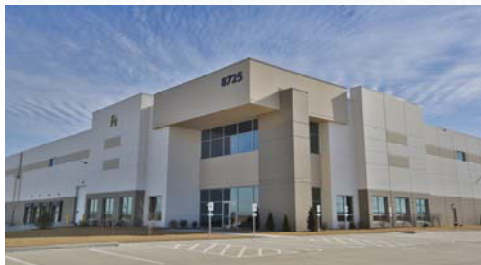
First Park 94 - Building II | Somers, WI
