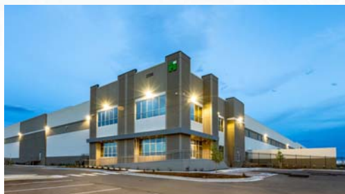
First Aurora Commerce Center - Building D | Aurora, CO
