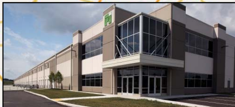
First Logistics Center @ I-83 20 Leo Lane York, PA
